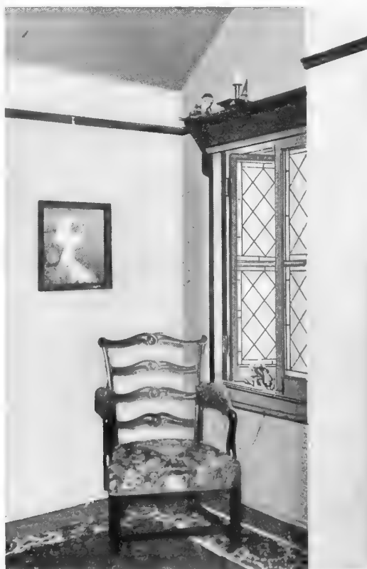
The Angle of the Room Shows the Line of the Roof Which is only Three and a Half Inches from the Inside of the Room to the Open Air
